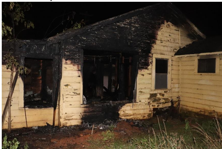
1446 Hamilton Road in LaGrange
