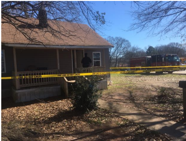
Location of fire on Reeves Street
