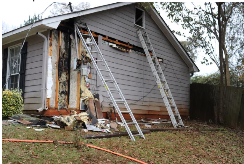
Structure Fire at 111 Daniel Court
